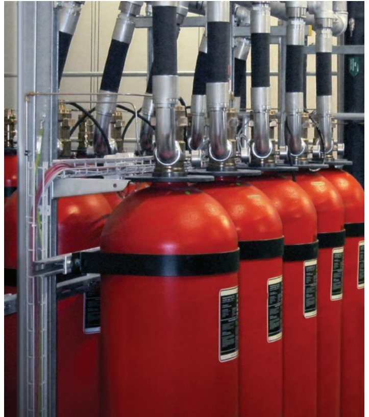
Viking Special Hazards can provide multi-cylinder and multi-zone systems to protect any special hazard area.
